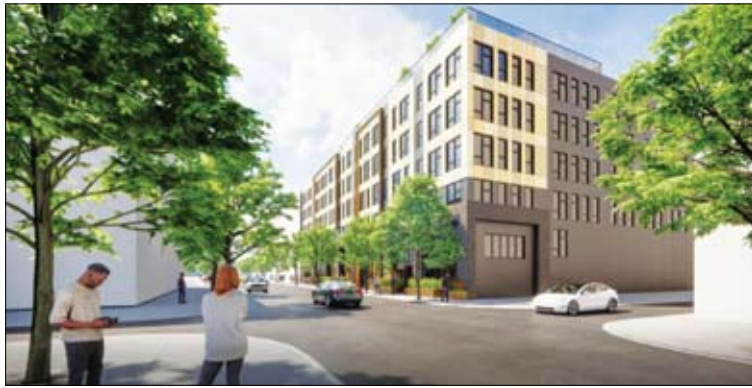
A new mixed-use building going up in a highly-congested area will feature a severe-shortage of off-street parking. Future residential and commercial tenants who own cars, but cannot secure parking, will find street parking difficult to secure.
