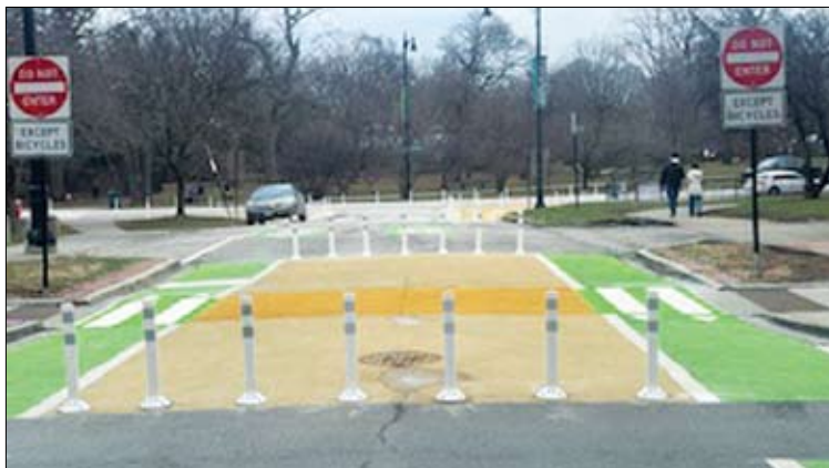
Dickens Dr. is now blocked at the intersection with Stockton. There are posted signs saying, "Do not enter except bikes." Chicago Park District employees can also use the block to park their cars on.
