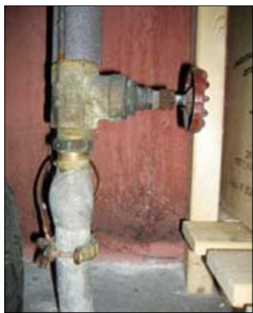
Lead service lines can be connected to the residential plumbing using solder and have a characteristic solder "bulb" at the end, a compression fitting, or other connector made of galvanized iron or brass/bronze.
