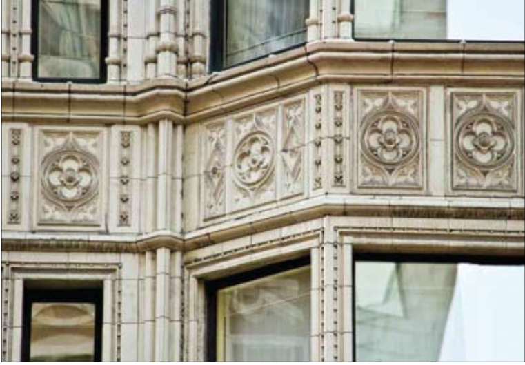
The gleaming terracotta façade of the 121-year-old Reliance Building is one of Chicago’s most highly-visible and most successful examples of architectural preservation and reuse.
