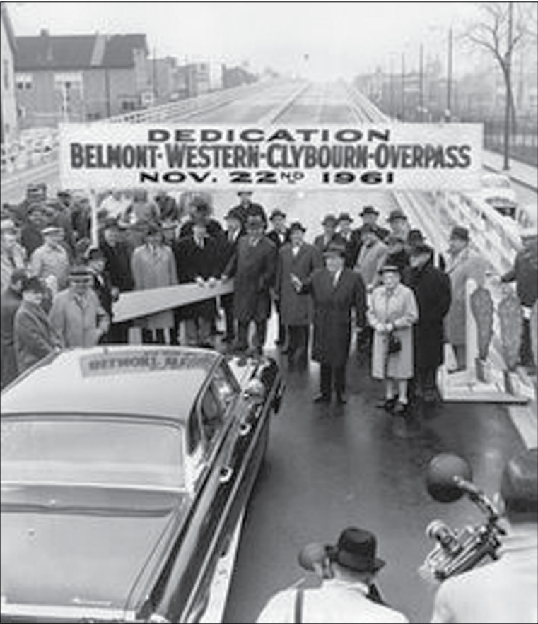
Mayor Richard J. Daley dedicating the Belmont and Western overpass in 1961. It was built to help reduce congestion in the area caused by the Riverview Amusement Park.
