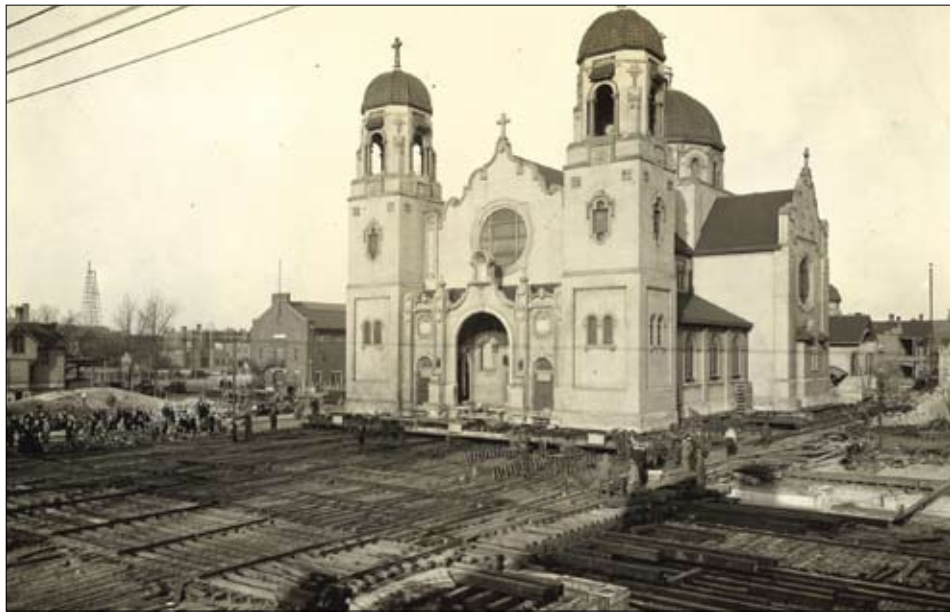
At one time, Our Lady of Lourdes Catholic Church occupied the current parking lot site. In 1929, in preparation for the Ashland Ave. street widening project, the pastor, Rev. James Scanlon helped to move the church across the street.
