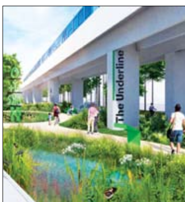
One possible use for space under the tracks is for rain garden swales that can help manage water.
