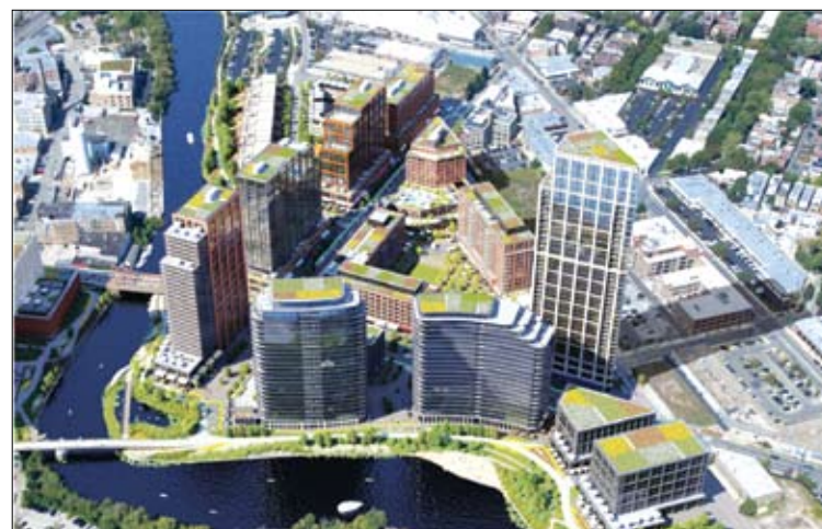
Foundry Park is what became of a portion of the Lincoln Yards development on the Chicago River.
