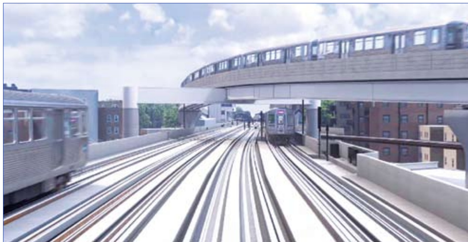
The new RPM Bypass is open for business. It will carry the Kimball-bound (northbound) Brown Line CTA trains over north-and southbound Red and Purple Line tracks just north of Belmont station.
