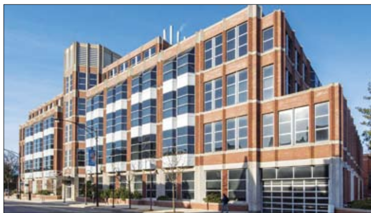
The 2430 N. Halsted building owned by Sterling Bay, that houses BioLabs, is situated in the heart of Lincoln Park and features state-of-the-art wet lab space. Image courtesy Sterling Bay
