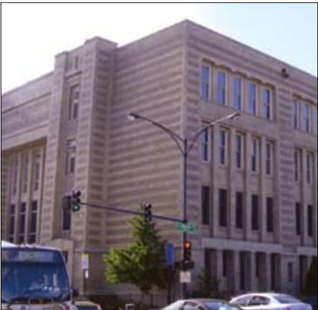
The former Trumbull school building at Ashland and Foster
