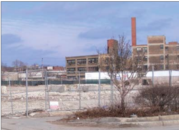
Here's all that's left of the Finkl Steel works. The 35-acre site is already attracting interest from all kinds of high tech, light industrial operations.
