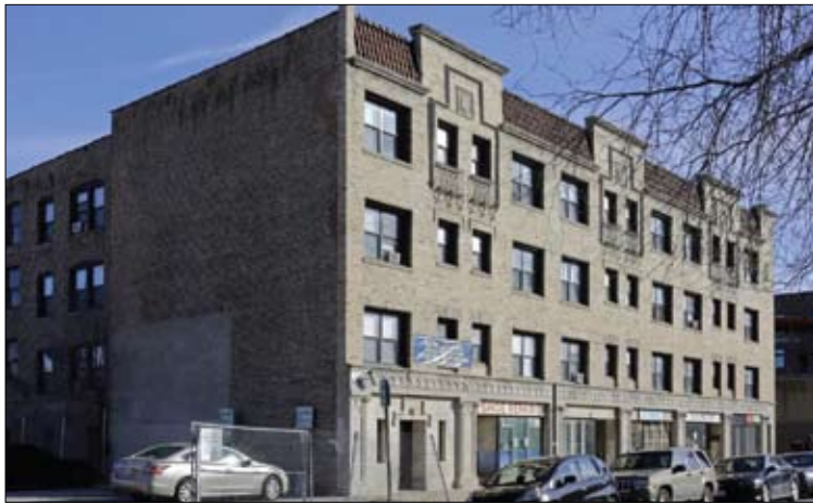
Loyola Univ. of Chicago purchased the property at 1226-1234 W. Loyola Ave. with plans to tear down the building once all the tenants vacated the site.
