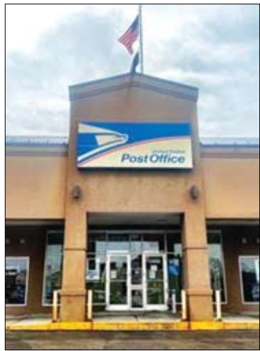
U.S. Post Office at 3024 N. Ashland Ave.
