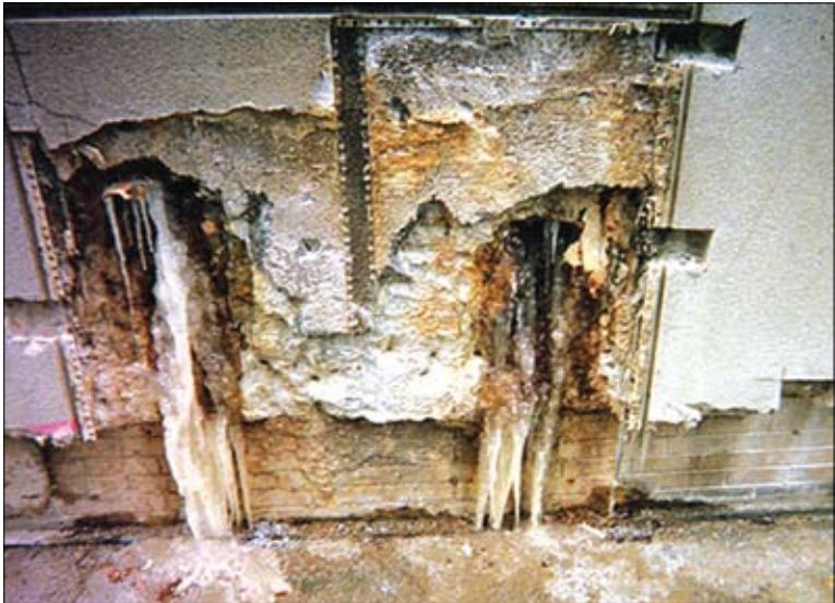
The base of an exterior wall at Hyatt Regency Chicago, seen here on Lower Wacker Dr. Water has flowed down the side of the building, frozen, and expanded, breaking off parts of the wall. Photo by David Sudler
