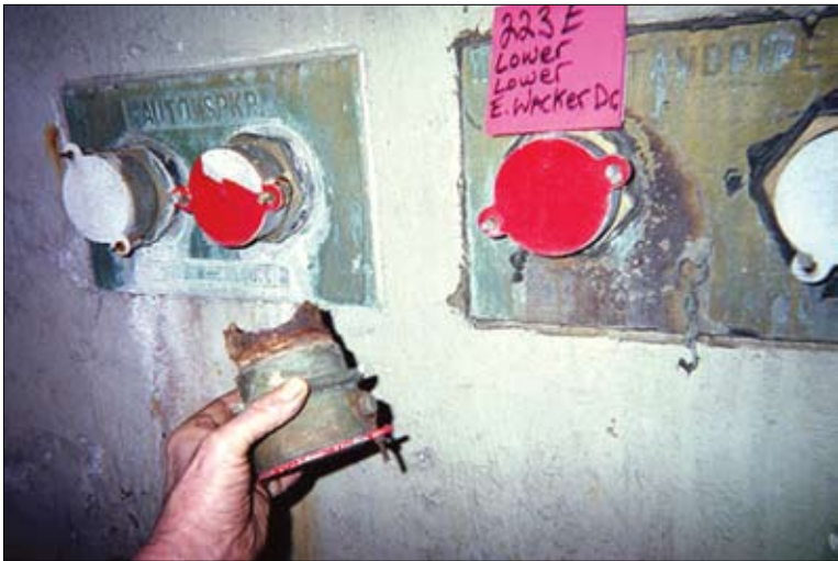
Broken and dirty standpipes at 223 East Lower Wacker Dr.
