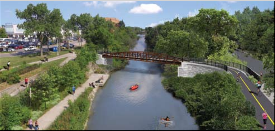
Last week the city broke ground on a new bike bridge in the West Rogers Park neighborhood called “Lincoln Village Pedestrian Bridge.”
