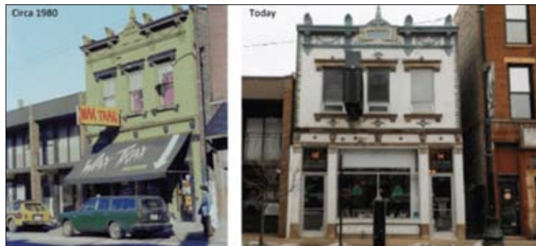
Wax Trax! before and after the green paint was stripped away, returning the building to its original exterior color.
