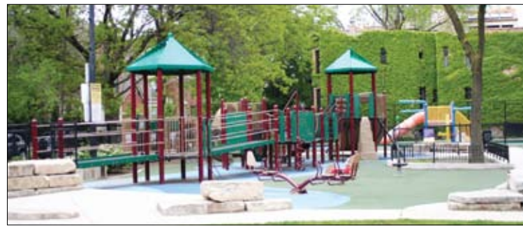
The water park at Adams Playlot in Lincoln Park, built 20 years ago, has deteriorated substantially and may not be repaired.
