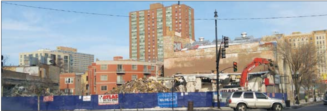
Uptown's City Sports building, 4601-4613 N. Broadway, has been demolished to make way for a new nine-story high density, 200-unit building.
