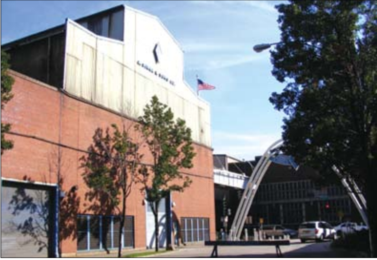
Demolition of the century-old Finkl Steel plant, once one of the area's largest and oldest employers, is scheduled to get underway this week.
