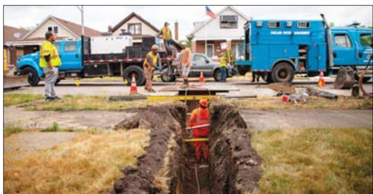
A construction crew completes a lead service line replacement at a Chicago home in June 2023. Courtesy Vanessa Bly/NRDC
