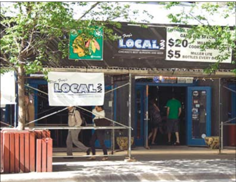
A condo association's construction scaffolds in front of the bar in their building last April.
