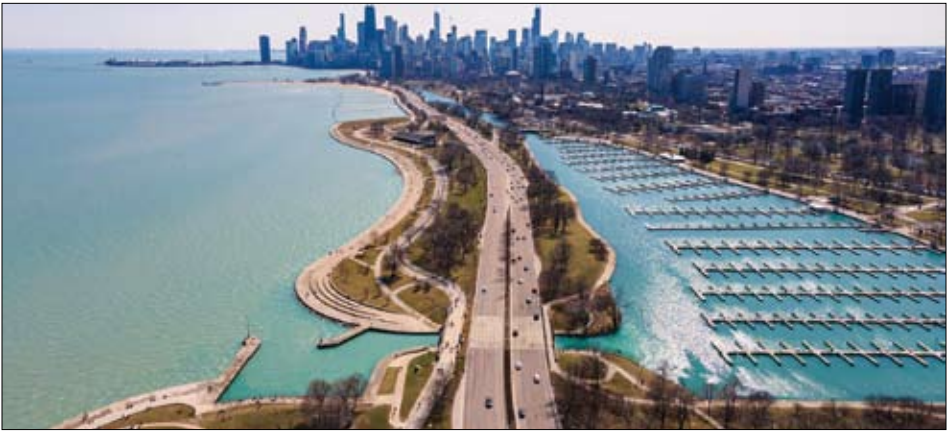
The highway engineers had very different priorities than the parks commissioners which is reflected in post-war changes to N. Lake Shore Drive.
