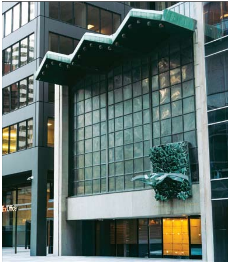
Chicago Loop Synagogue, a 2026 Chicago 7 Most Endangered. Chicago Loop Synagogue, 1957, Loeb, Schlossman & Bennett, 16 S. Clark St. Photo courtesy Lily Ma / Numi Studio
