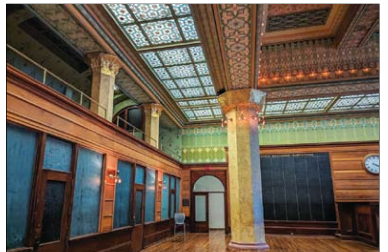
The Chicago Stock Exchange Trading Room, a 2026 Chicago 7 Most Endangered. The Chicago Stock Exchange Trading Room, 1894 Dankmar Adler and Louis Sullivan, dismantled in 1972 and reconstructed 1977 Vinci-Kenney Architects, 111 S. Michigan Ave. Photo courtesy Eric Allix Rogers
