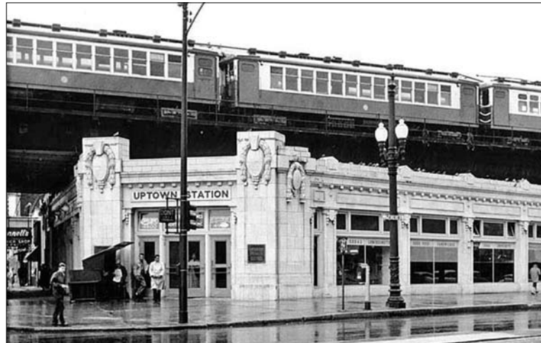
The Arthur Gerber-designed Uptown Station building is seen here in 1959, looking westward on Wilson and north on Broadway. Image courtesy CTA
