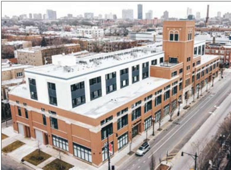
The former Sears Store site spans an entire block of Lawrence Ave.
