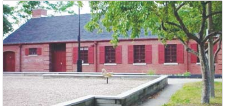
Originally built as a comfort station, which included showers and bathrooms, the current Emmerson Park Fieldhouse only allows for limited programming and is in need of a major rehab.
