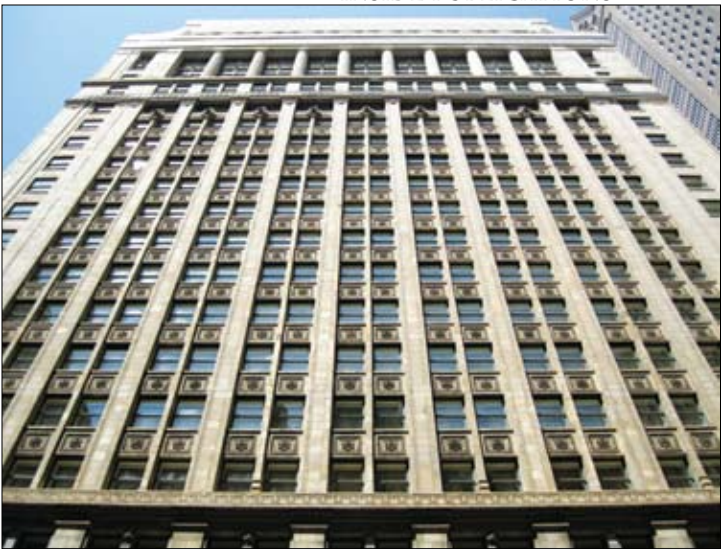
Continental and Commercial building, 208 S. LaSalle St.
