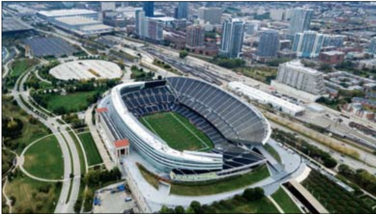
The latest $2-billion to $4-billion trial balloon is being floated by the Chicago Bears, who want taxpayer help in building a new, grandiose domed stadium on the parking lot just south of Soldier Field.
