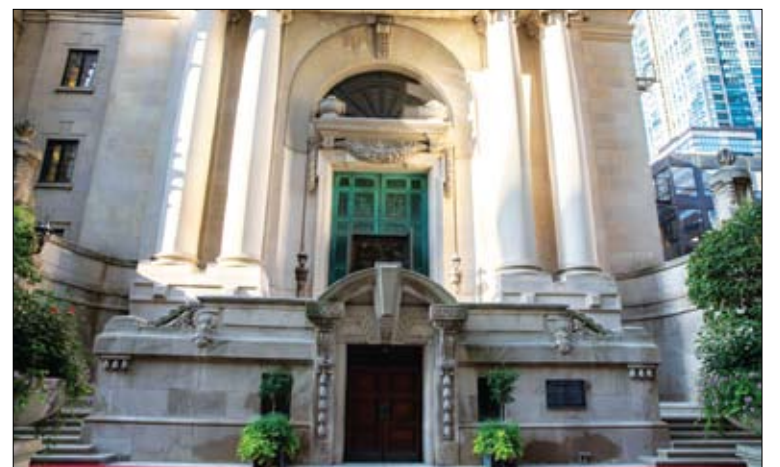
The Commission on Chicago Landmarks may soon tap the John Murphy Memorial Building, 50 E. Erie, as Chicago's next landmark building.
