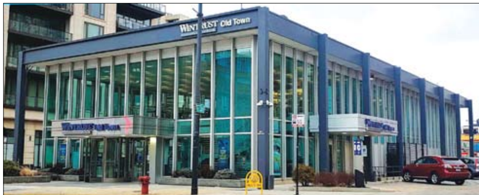
Preservation Chicago considered the former North Federal Savings Bank (Wintrust Bank) Building at 100 W. North Ave., a "Midcentury Modern gem." Photo courtesy Adam Natenshon
