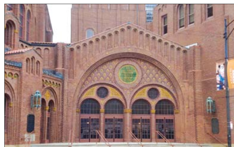
[Top] The Archway Standard Station/BP Service Station, 1647 N. LaSalle Dr. (Georg Terp, 1971) is now considered to be an at-risk landmark by Preservation Chicago, as is the Moody Memorial Church [bottom], 1635 N. LaSalle Dr. (John Fugard of Fugard & Knapp, 1924-1925).
