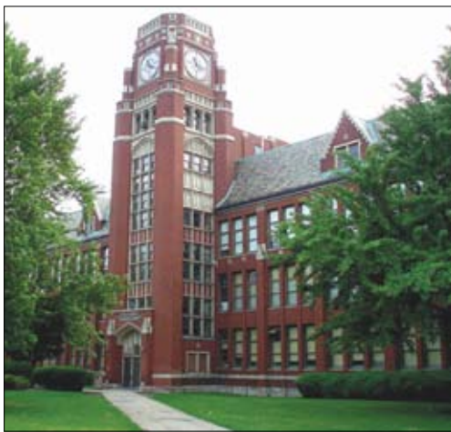
A $50-million renovation of Lane Tech College Prep High School, 2501 W. Addison St., is scheduled to begin April 1 and continue through early 2017.
