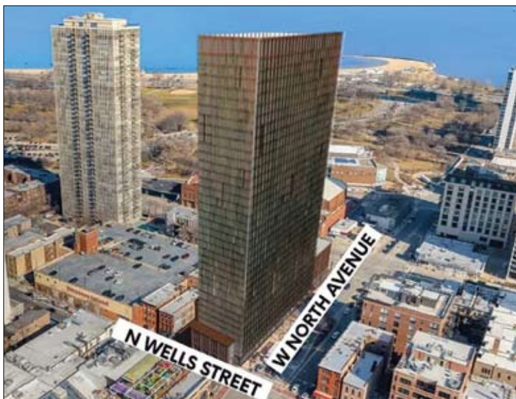
Developers Fern Hill hosted an online virtual community meeting March 21 regarding the proposed high-rise at 1610 N. LaSalle Dr.
