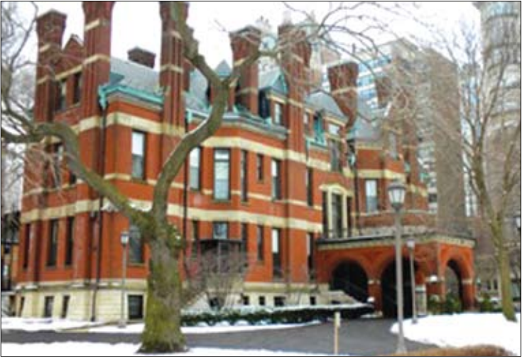
The Cardinal's Residence now empty and ready for reuse is the final rest for Constable Quinn.
