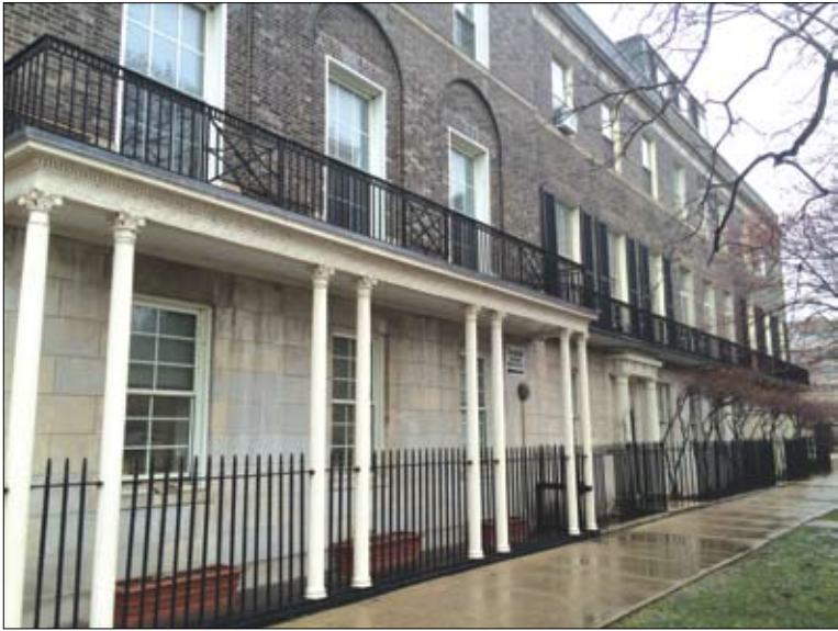
For about 40 years, the Row House located at 2700 N. Lakeview (the largest) was operated as the Dincin Center, a facility of the Threshold's social-services agency.
