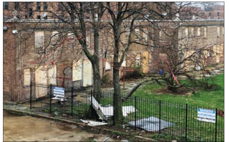
After a decade of neglect by the Chicago Housing Authority, the long-stalled redevelopment of the southern section of the Julia C. Lathrop Homes south of Diversey Pkwy. at Damen Ave. may finally occur if the Chicago City Council passes legislation. The riverfront property has been a community eyesore since they moved residents out starting in 2009.
