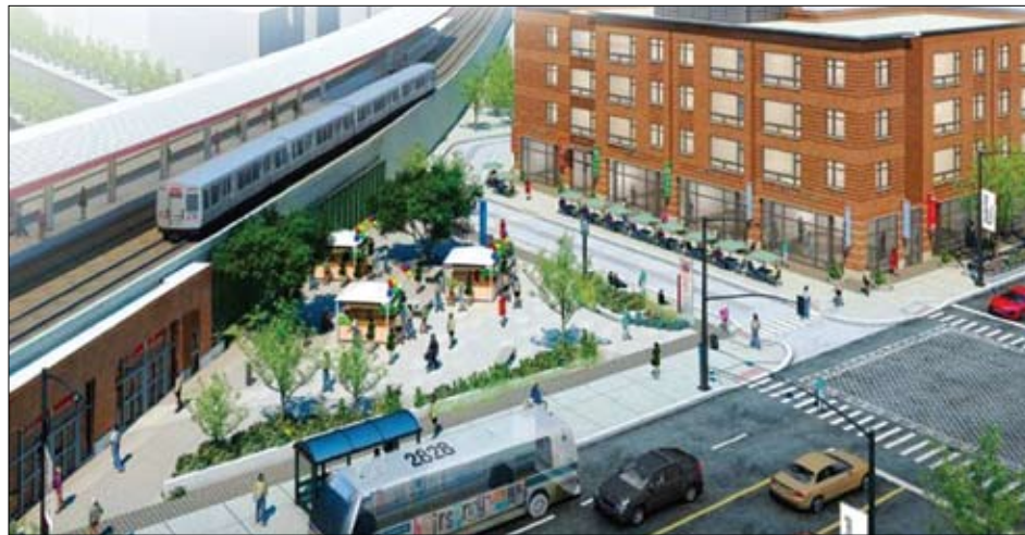
The RPM modernization plan may enable train access in both directions rather than access that differs by direction of travel. The Loyola Stop platform would also be lengthened to accommodate 10-car trains.
