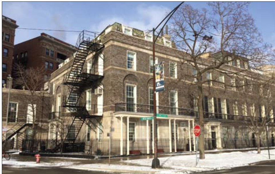
"The three-story row houses were built with steel posts, reinforced concrete, and concrete and hollow clay-tile floors and walls, substantial and expensive materials that at the time were more common to larger commercial buildings and apartments than to private homes," according to a report released by city officials last Wednesday.
