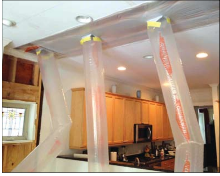
The handyman opened the family room ceiling, found the leak, and traced it back to the shower wall between the bath and master bedroom. After that wall was opened, the plumbers quickly repaired the broken copper pipe. But now the house had to be dried out with blowers.
