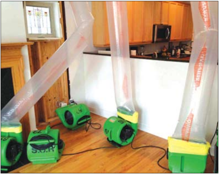
The handyman opened the family room ceiling, found the leak, and traced it back to the shower wall between the bath and master bedroom. After that wall was opened, the plumbers quickly repaired the broken copper pipe. But now the house had to be dried out with blowers.
