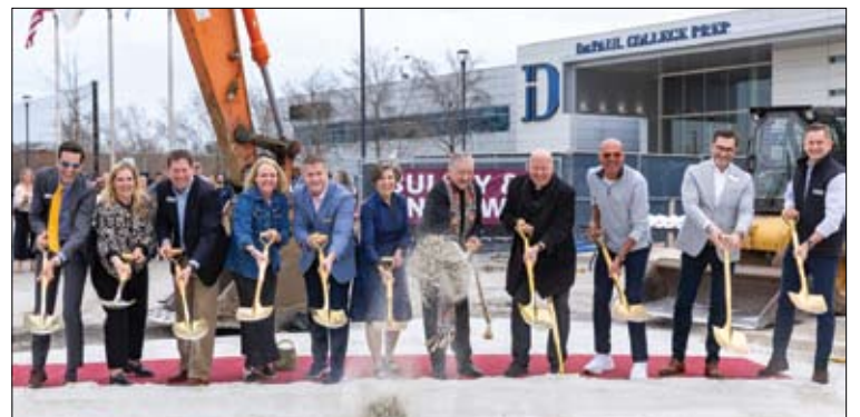
Cardinal Blase Cupich, DePaul Prep President Mary Dempsey and others at the ground breaking of DePaul Prep's new athletic facility.
