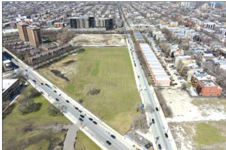
New CHA redevelopment site at 1450 N. Larrabee St. looking north. Photo by CST Tyler Pasciak LaRiviere
