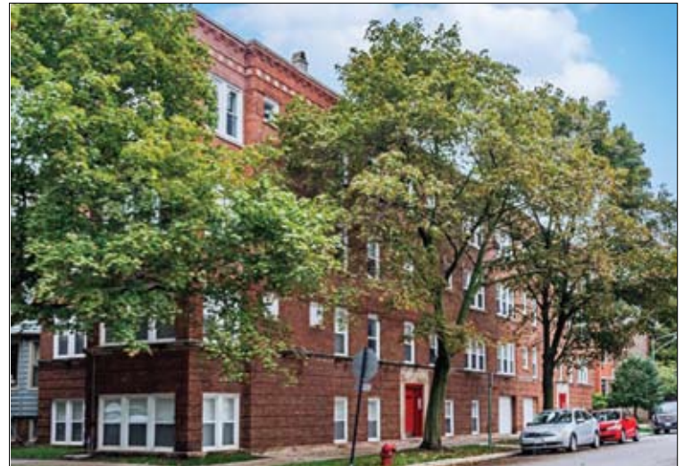
These trees may now be on death row now so that century-old water lines below them and in need of repairs can be replaced.
