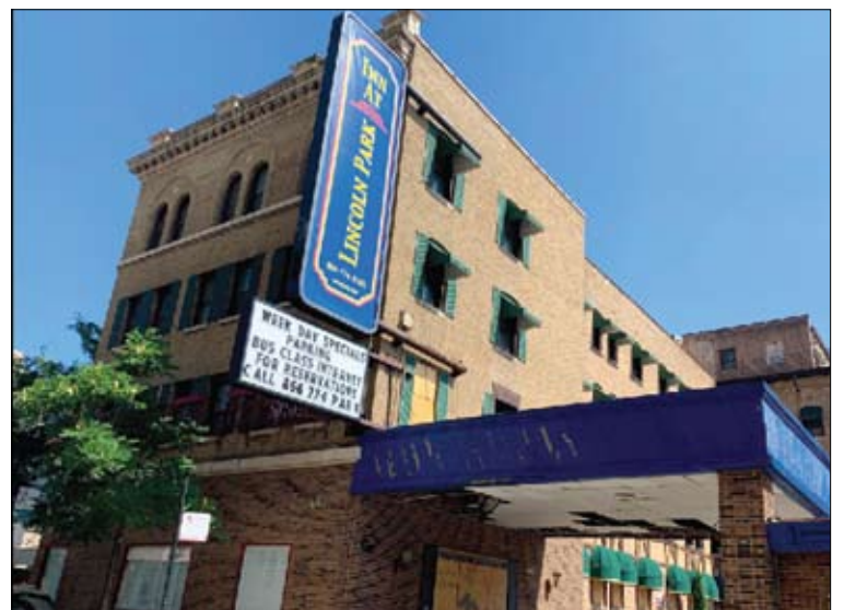
The century-old former Inn at Lincoln Park, 601 W. Diversey, may soon be under construction.
