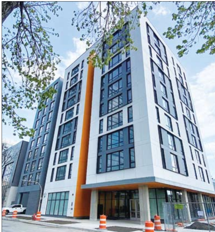
The 10-story Post Chicago, 853 W. Blackhawk St., is located next to Chicago's second-largest retail district, the Clybourn corridor.
