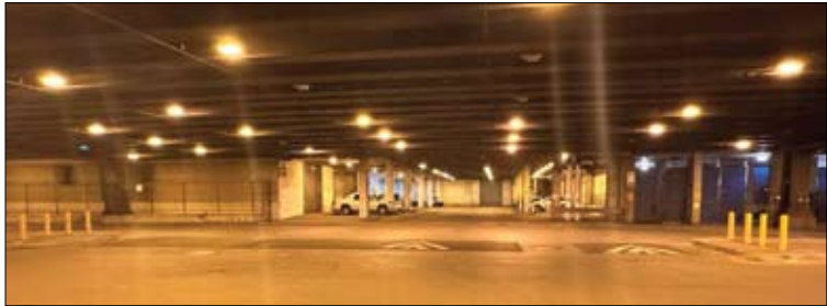
Newly-installed bollards, concrete islands, and speed humps are designed to stop donut-spinning sideshows at Columbus and South Water. Photo courtesy of Ald. Brendan Reilly
