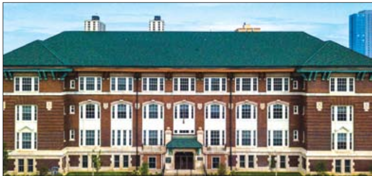
In 2013, the Chicago Public Schools closed the Stewart School at 4525 N. Kenmore Ave., along with 48 other public school buildings.
