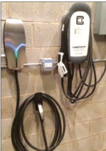
The Tesla 80A Wall Connector.
