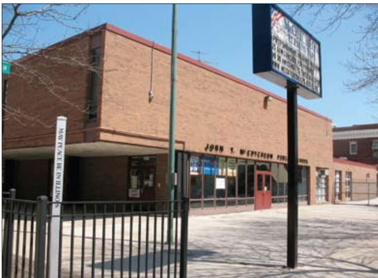
McCutcheon Elementary School is one of only five schools in Chicago's 500-school district without its own gymnasium.
