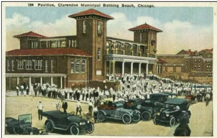
Work on the new Clarendon Park Fieldhouse [top] began in 2022. The $13 million makeover will be unveiled late fall or early winter. A 1916 image [bottom] of the beachfront Clarendon Park bath house, of which the new fieldhouse today occupies.
