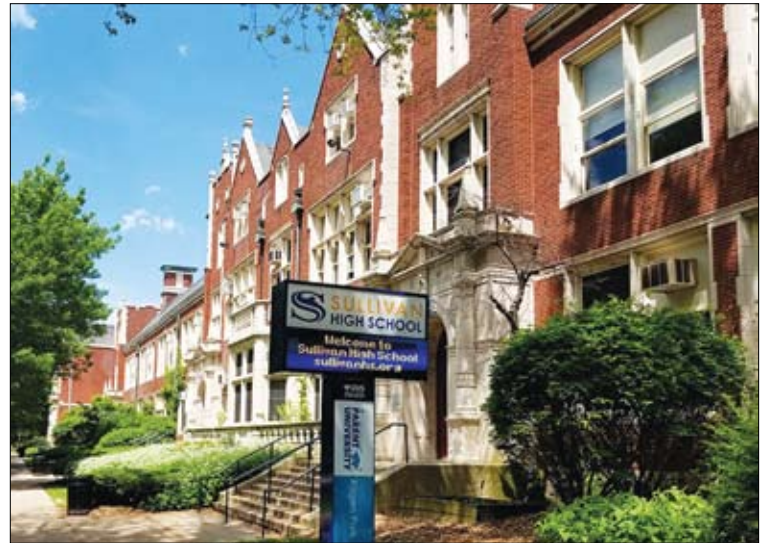
Sullivan High School, 6631 N. Bosworth Ave., is under construction.
