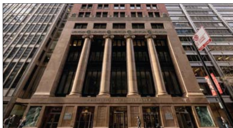
The former Harris Trust & Savings Bank building, 111 W. Monroe.
